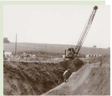
Sewer pipe installation, 1960.
